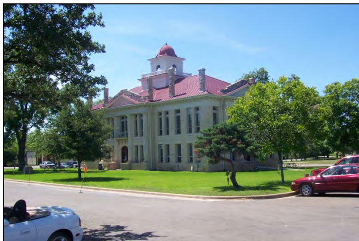
Figure 4. A Rural Courthouse Square: Johnson City, TX (Source: Dumbaugh).
