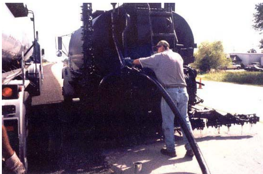
Figure 5-5. Transferring Asphalt from Transporter to Distributor.
