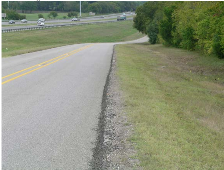
Figure 3-8. High Edge Resulting in Pavement Edge Corrosion.
