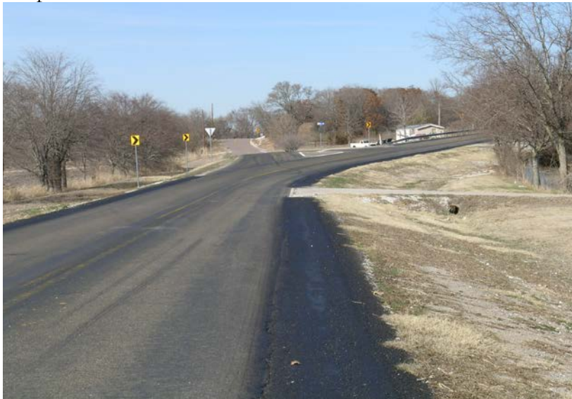
Figure 3-10. Edge in need of repair and fog seal.
