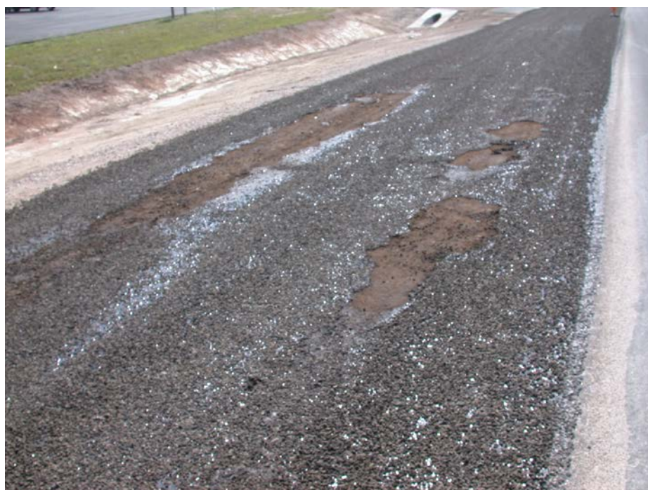
Figure 1-4. Construction Traffic Causing Delamination of Surface Treatment from Granular Base Course.
