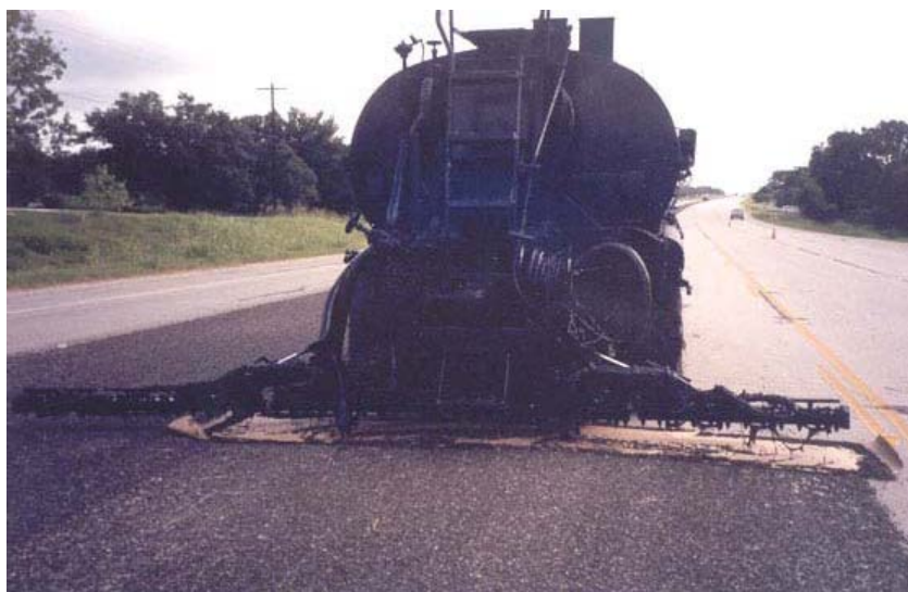
Figure 5-6. Correct Starting Position over Paper Joint.
