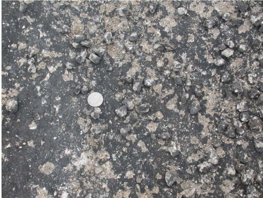
Figure 1-19. Failure of Prime Coat Due to Loose Rock on the Road.
