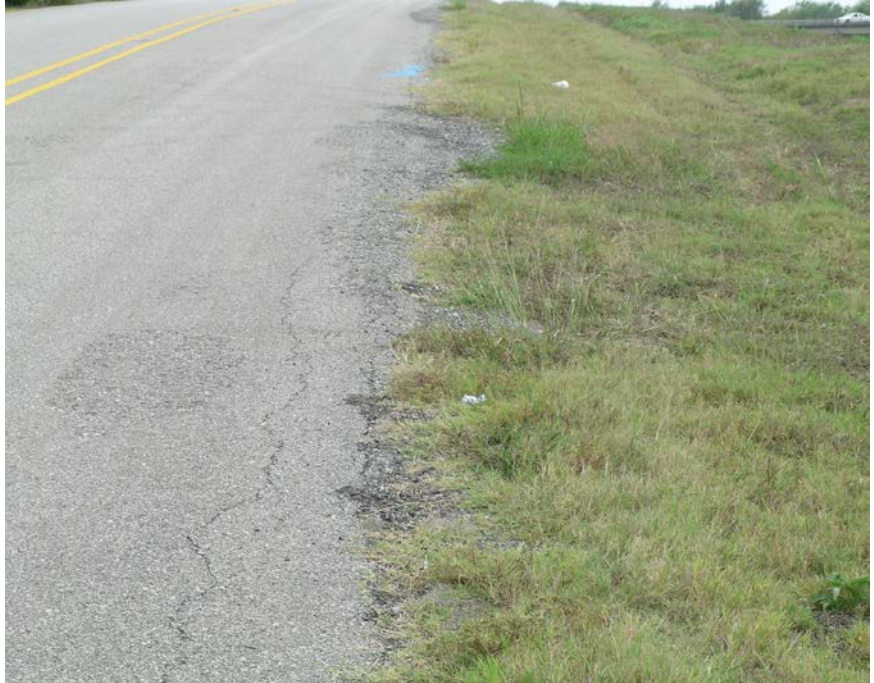
Figure 3-7. Surface deterioration due to encroaching vegetation.
