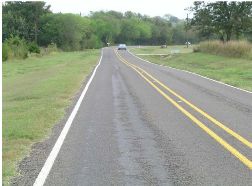
Figure 3-11. Aggregate Loss Due to Fresh Patches.
