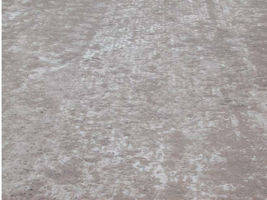
Figure 1-10. Flexible base surface finished using trimmer and ready for prime coat application.
