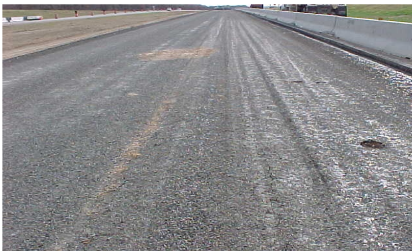
Figure 1-15. Curing Flex Base.
