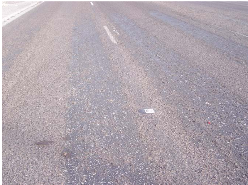
Figure 1-22. Seal Coat Pavement Surface Exhibiting Aggregate Loss.
