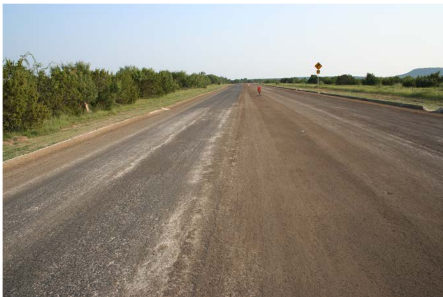
Figure 1-18. Failure of Prime Coat Before Surface Treatment is Applied.
