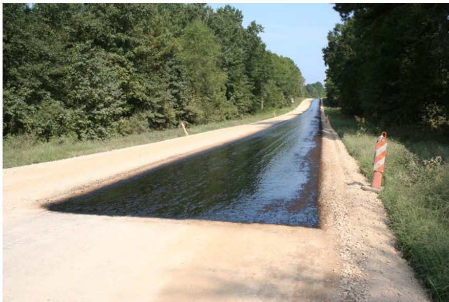
Figure 1-12. Spray Prime (MC-30, AE-P).
