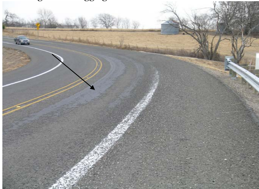
Figure 3-12. Shelling Rock from Fresh Patch.
