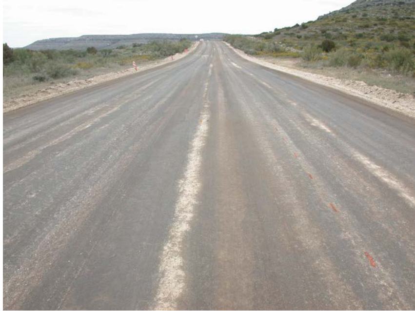
Figure 1-17. Wearing of Prime Coat by Traffic.
