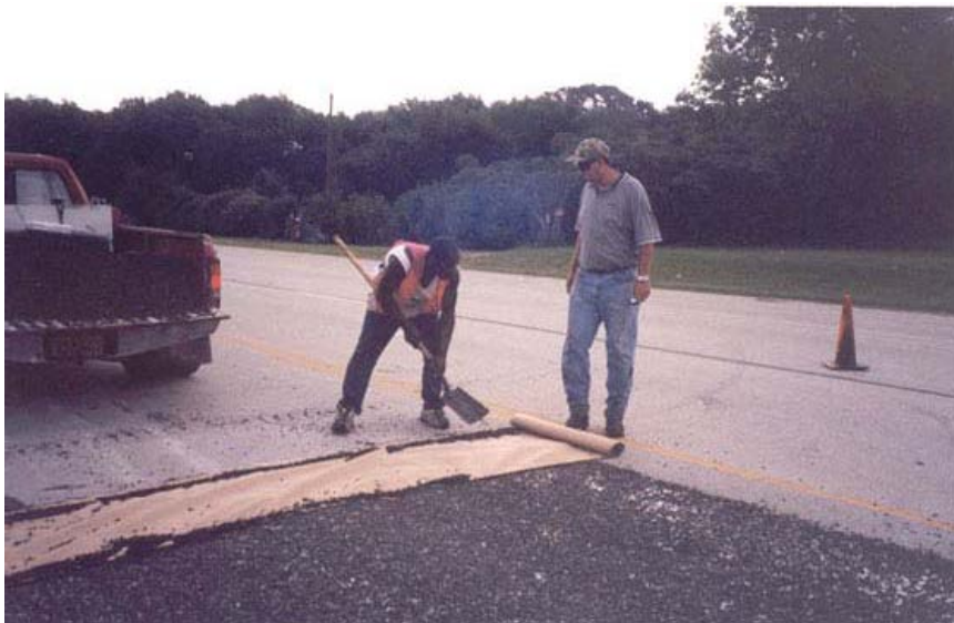
Figure 5-3. Placing a Paper Joint at Beginning of Shot.
