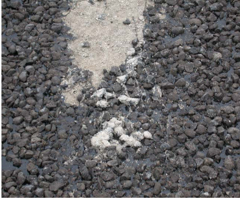
Figure 1-20. Pick-up of Prime and Surface Treatment by Construction Traffic.
