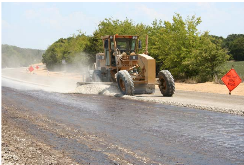
Figure 1-13. Worked-in (Cut-in) Prime.
