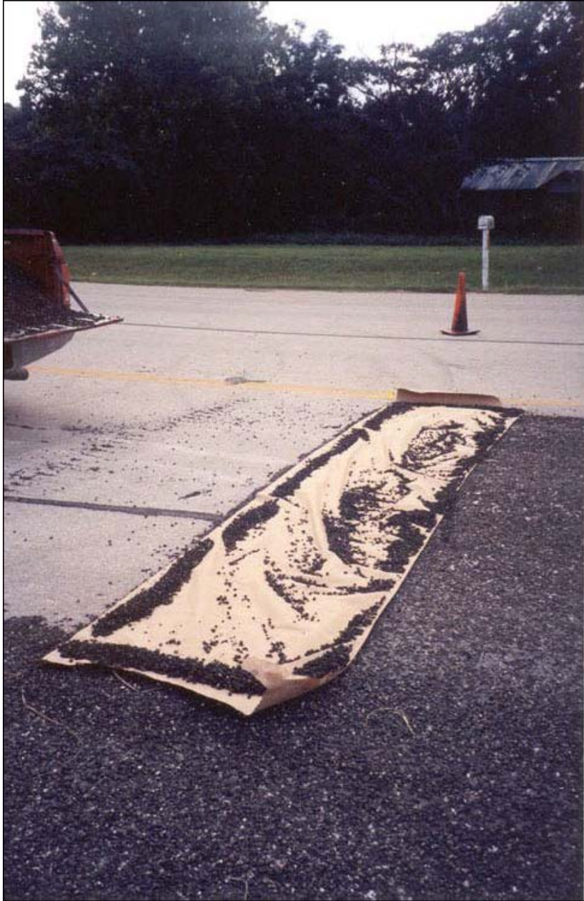
Figure 5-4. Paper Joint in Place at Beginning of Second Shot.
