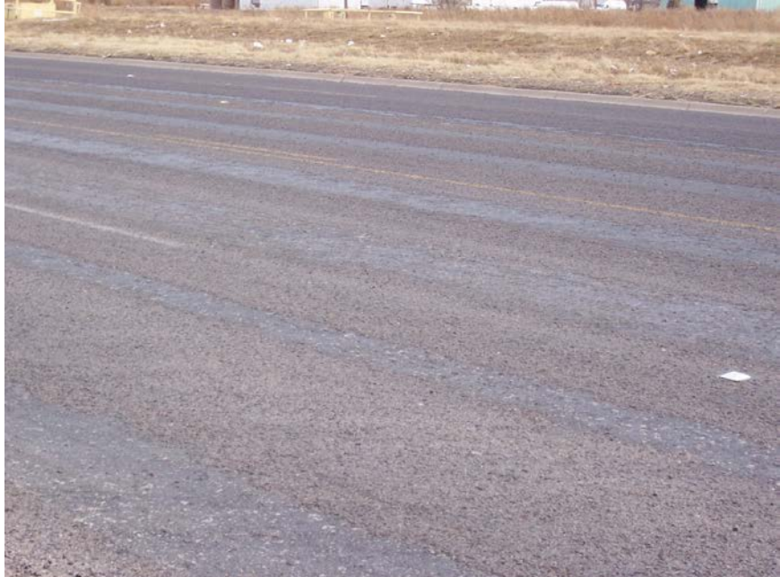
Figure 1-21. Seal Coat Pavement Surface Exhibiting Aggregate Loss.
