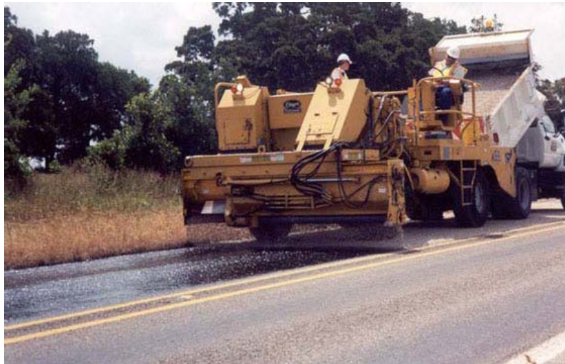
Figure 4-27. Aggregate Spreader or Spreader Box.
