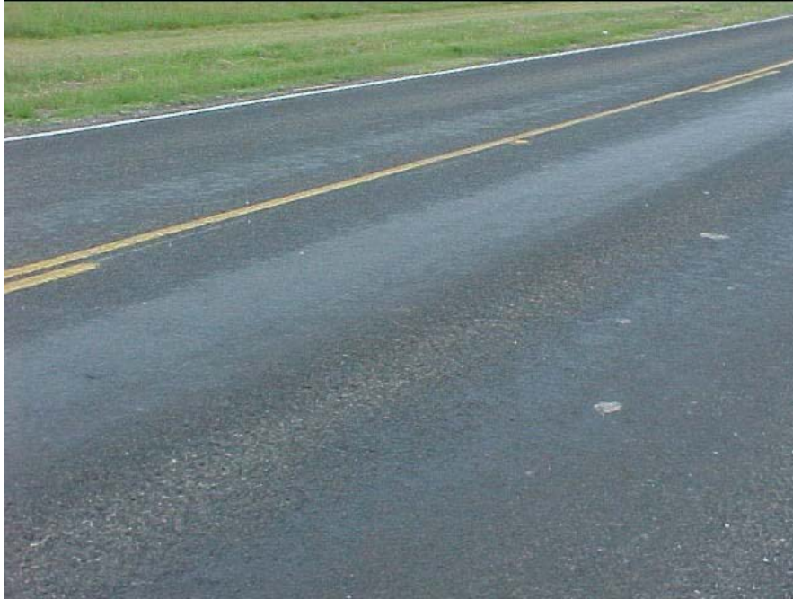
Figure 1-24. A Seal Coat Pavement Surface Exhibiting Flushing in the Wheelpaths.
