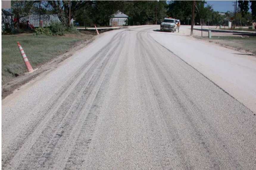
Figure 1-14. Covered (Inverted) Prime.
