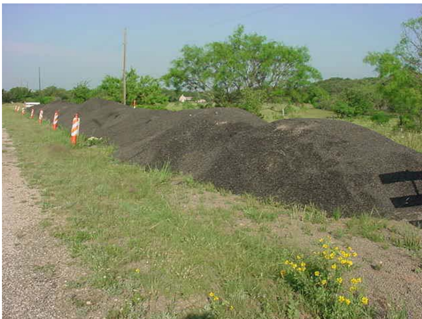
Figure 3-15. Properly Placed Aggregate Stockpiles.
