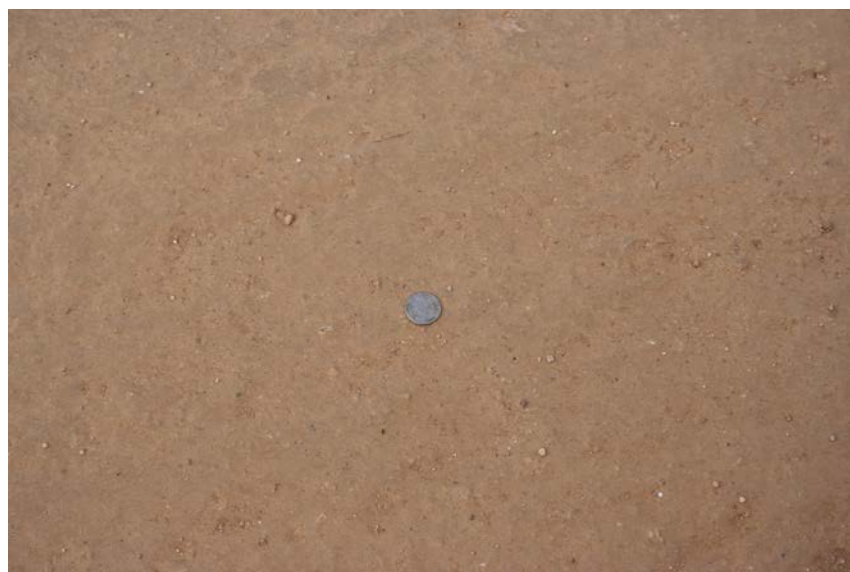
Figure 1-6. Finished Limestone Flexible Base.
