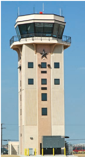
The new air traffic control tower at Mesquite Metro Airport. The 80-foot tall tower is staffed by Federal Aviation Administration contract air traffic controllers and will enhance the safety of the airport's daily operations.
